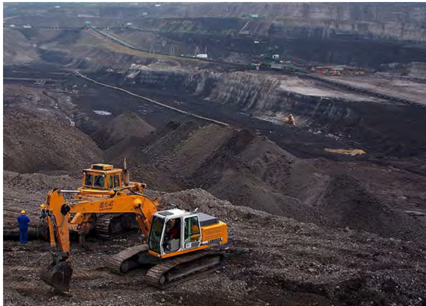
Plate 2 – Typical Open Cut
